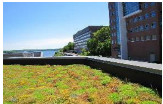
Example of extensive green roof
